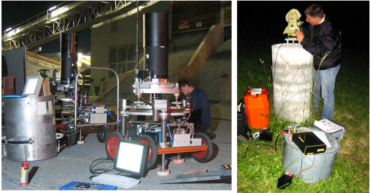
Figure 9, 10: Deployment of the two systems DIADEM (left) and TZK2-D on the AlpTransit construction site Bodio, summer 2005. Right picture: Measurement of an astronomical azimuth at the portal pillar Faido by means of the on-line measuring system ICARUS of ETH Zurich.
